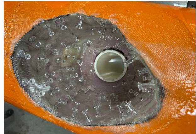
Figure 7: Push pins are used for the first layer to ensure good contact with the sides of the hole.
